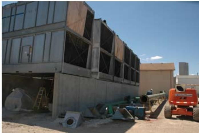
(Left) The six cooling towers have been installed and workers are preparing to connect the lines that run to the refrigerant condensers on the chillers.
