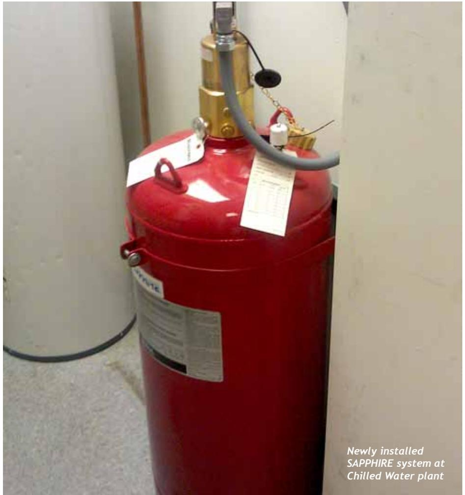
Newly installed SAPPHIRE system at Chilled Water plant
