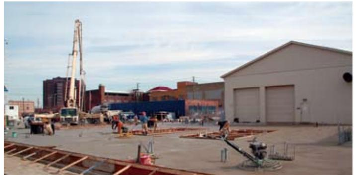
*Crews for Citizens Thermal Energy lay concrete for the expansion of the Illinois Street Chilled Water Plant.*
