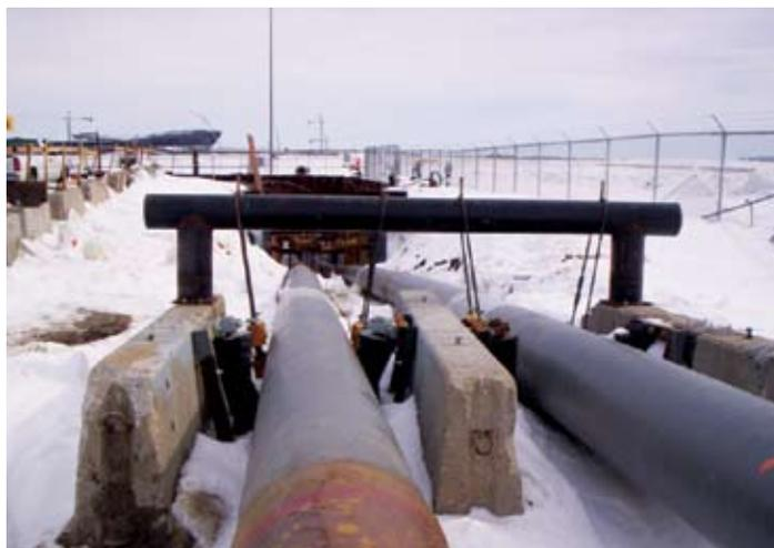
*Pre-insulated high temperature water pipes are being installed for the new Midfield Terminal.*
