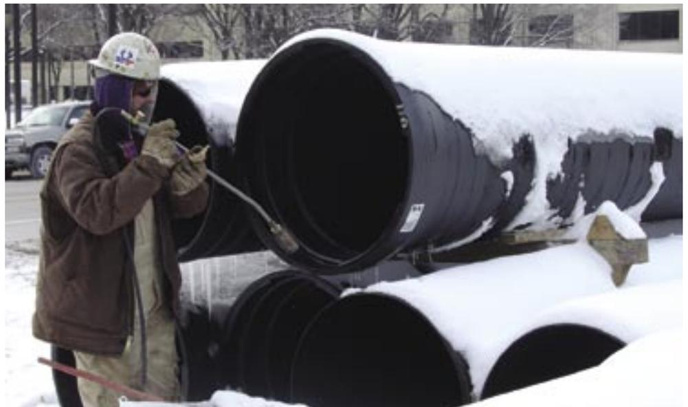
*A worker uses a torch to thaw ice that has formed on a section of iron pipe for the chilled water expansion.*
