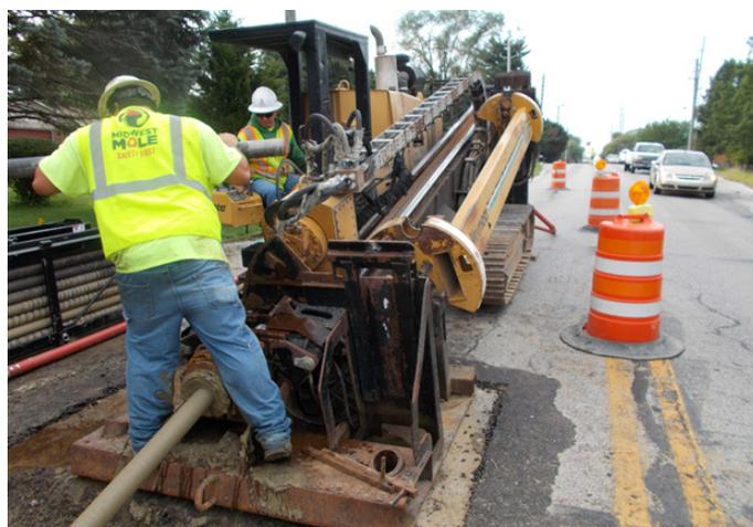
*During construction of the force main, you will likely see a drill rig (pictured above), pipe laid out on the road and traffic control devices.*
